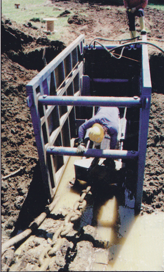
The 200-ton pipe burster used a maximum of 60 tons of pulling force throughout the project.
