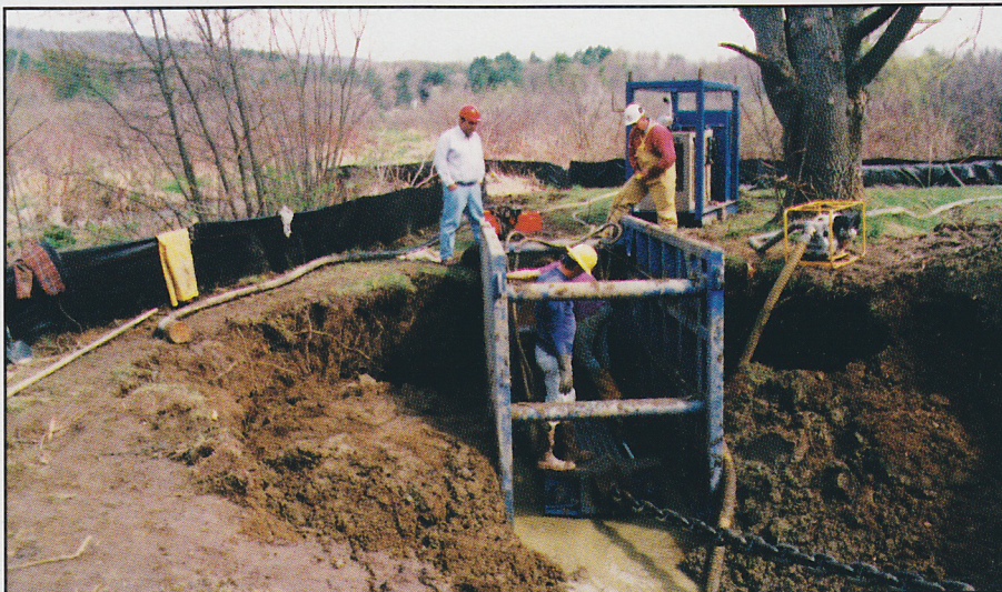
The pipe bursting unit makes a record pull in Stockbridge, Mass.
